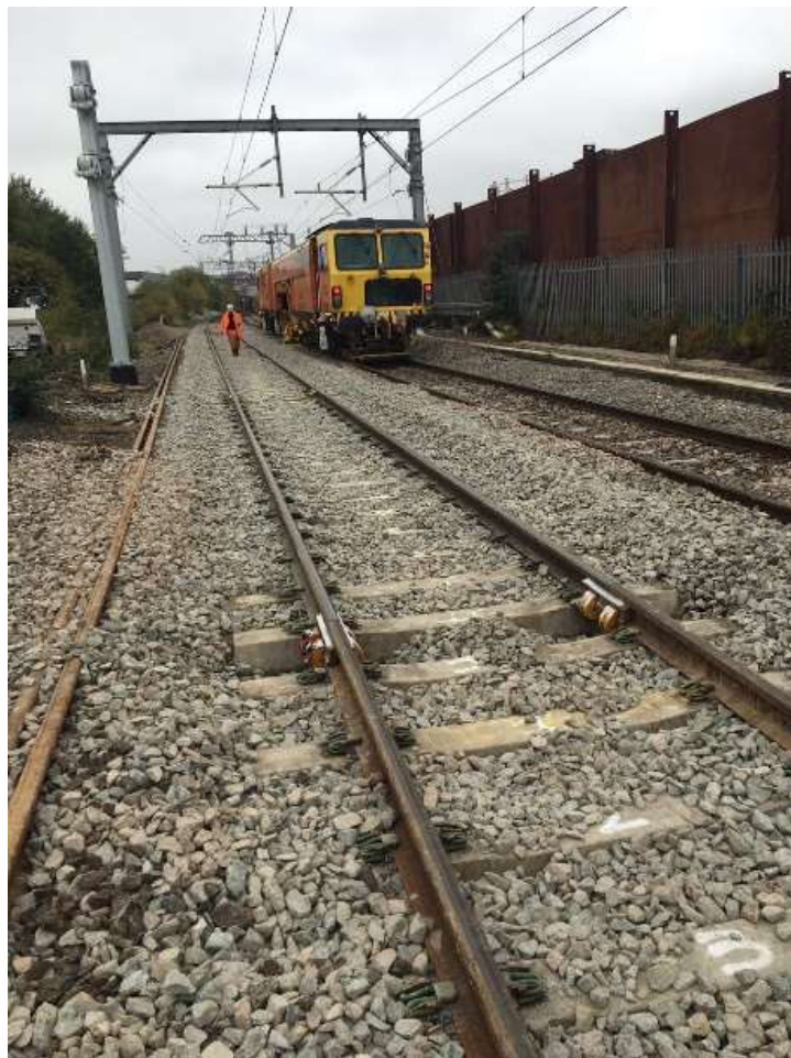
Figure 9: Tamping work on the railway track crossing Chat Moss. Over time, railway tracks settle with the passage of traffic; this is more likely to happen where the track passes over soft ground. The track may not settle evenly, resulting in track deformation. Tamping (i.e. packing - or tamping - the track ballast under the tracks) makes the tracks more durable, thereby ensuring good track alignment, smooth running and also preventing derailment.
