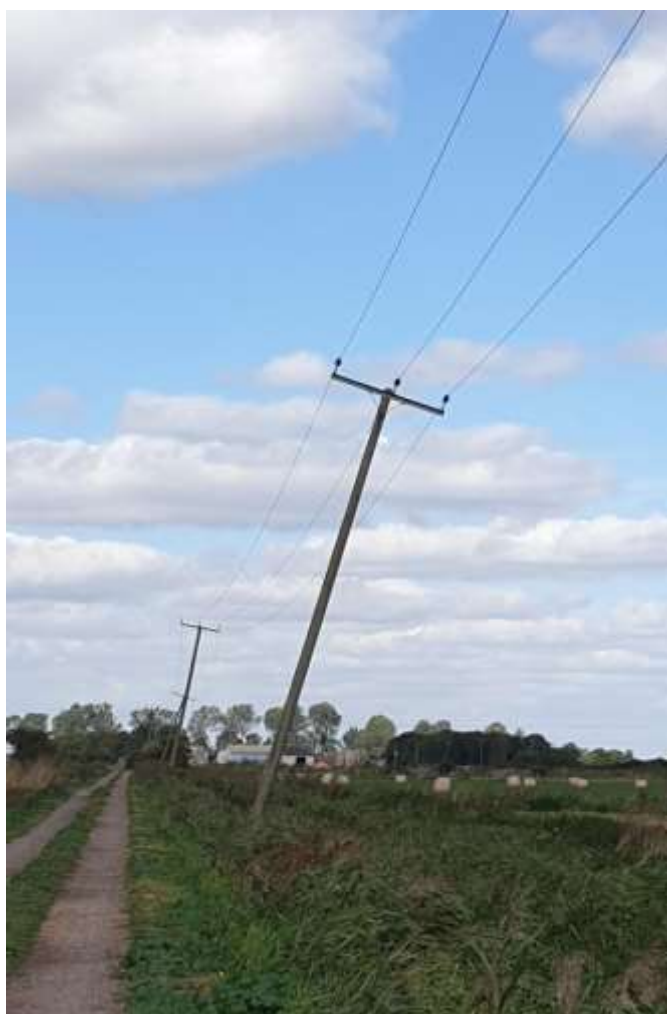
Figure 12: Subsidence damage to telegraph poles crossing drained peatland near Holme Fen, Cambridgeshire. (Photo – S. Page)
