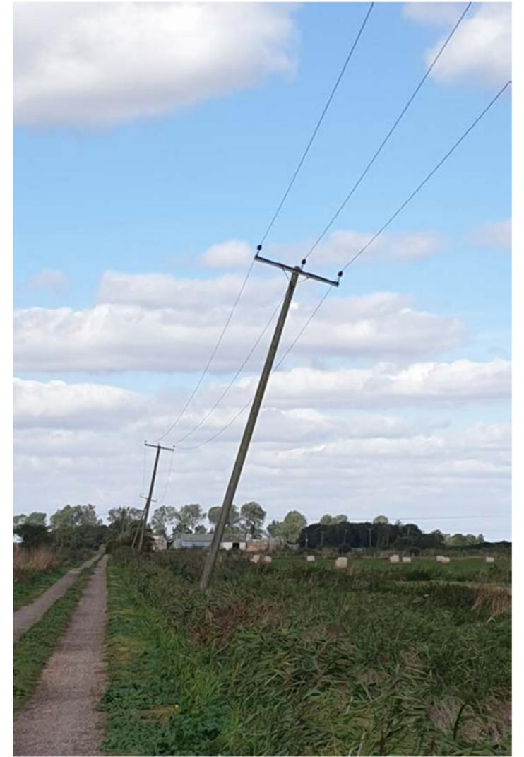
Figure 4: Subsidence damage to telegraph poles crossing drained peatland near Holme Fen, Cambridgeshire. (Photo – S. Page)
