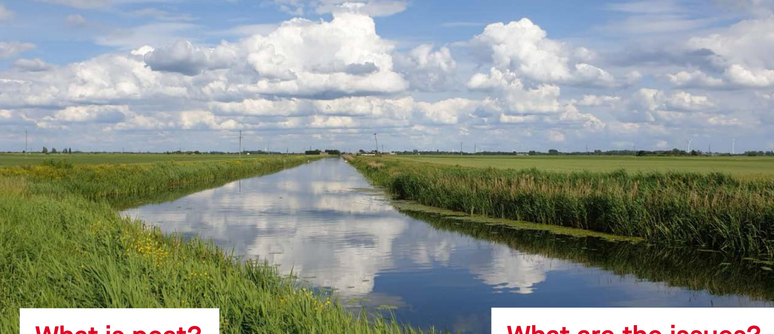
Figure 2: The Twenty Foot River (Drain) near Whittlesey was constructed in the mid-17th century. Water is pumped 'up hill' into rivers from the lower drains to protect agricultural land and settlements from flooding. (Photo - S. Page)
